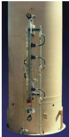
after the replacement
